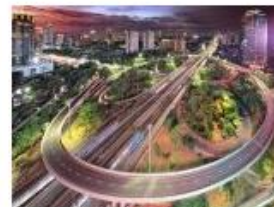
New Semanggi Fly Over
